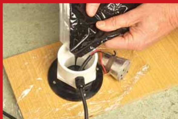
Photo 12: once mixed, cut the corner of the bag off and pour just a small amount – say a couple of millimetres or so – into the transducer housing. Put the bag to one side for a moment (remember to keep the pouring hole up).
