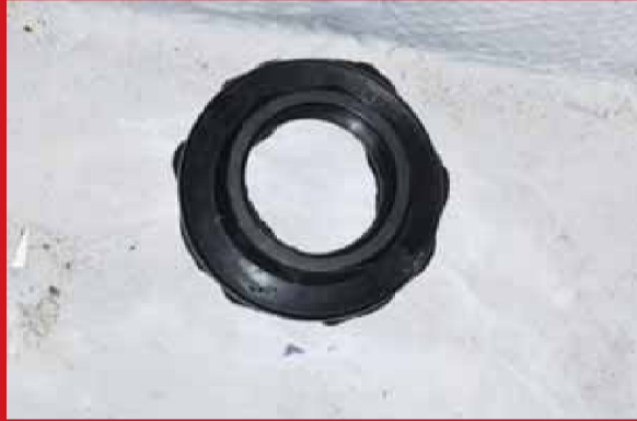
Photo 22: it's almost inevitable that there will be some J-B Weld oozing out from under the flange as you press it in place. The secret is to apply only as much pressure as is really needed to ensure the glue spreads right around, then wipe any excess off before it sets.
