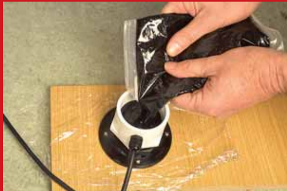
Photo 14: squeeze the potting compound out like toothpaste – not too fast, to be sure you don't get any bubbles trapped. Fill to a millimetre or so below the top of the tube – as it cures, it warms and expands. We found we used most of the 250g pack of resin.
